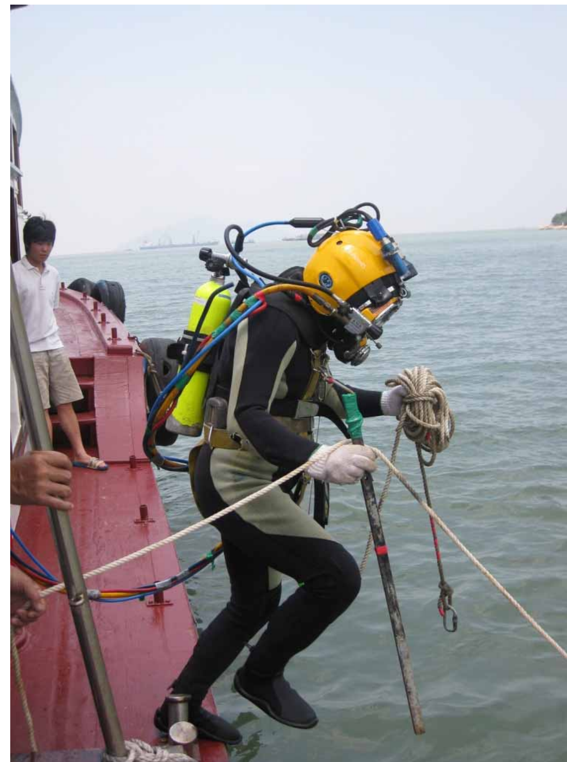
Diver entering water with metal probe and rope for circular search
